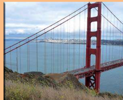
Golden Gate Bridge – San Francisco
